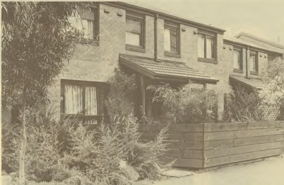
Some of the Victorian Housing Commission's new terrace homes in Fitzroy.
