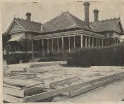
Carinya during renovations.
