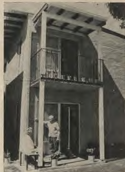
Keble Court, a block of flats runs by the Brotherhood in North Fitzroy.
