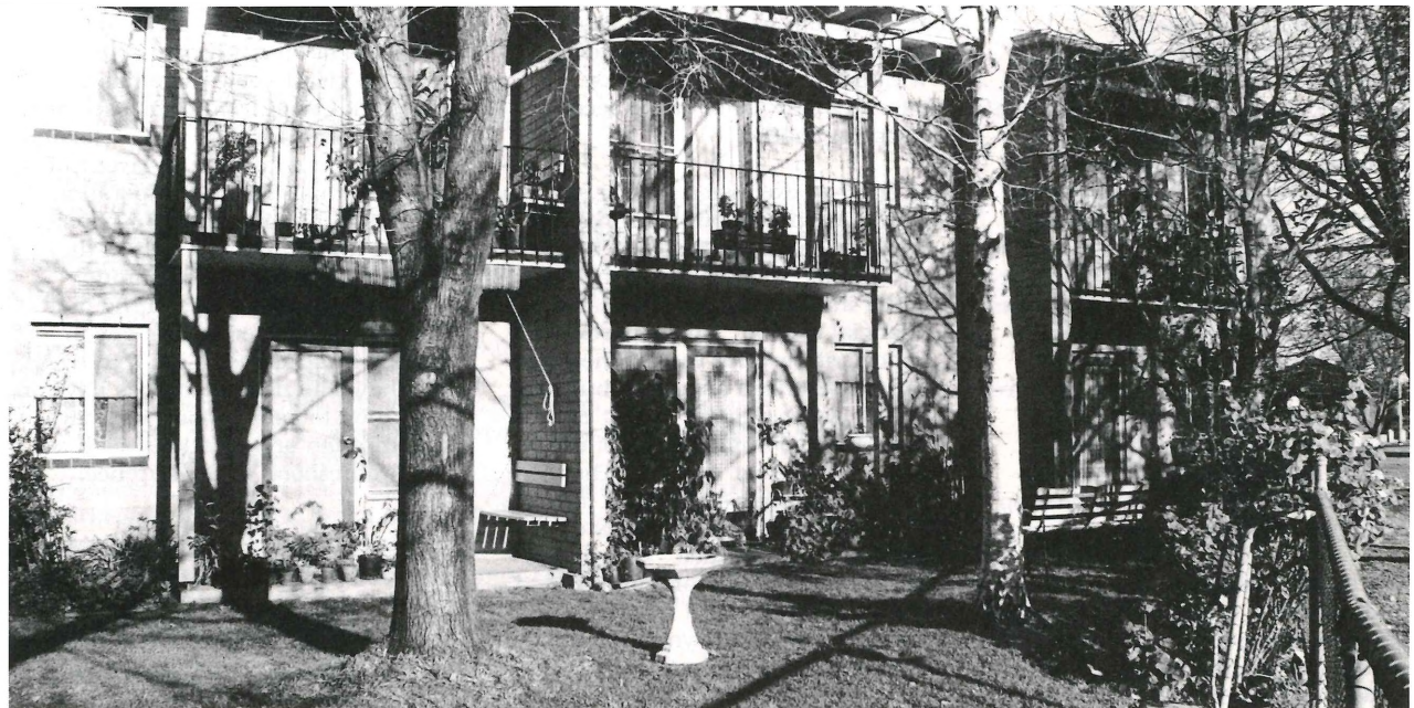
Keble Court, 30 units in Brunswick for the low-income aged.
